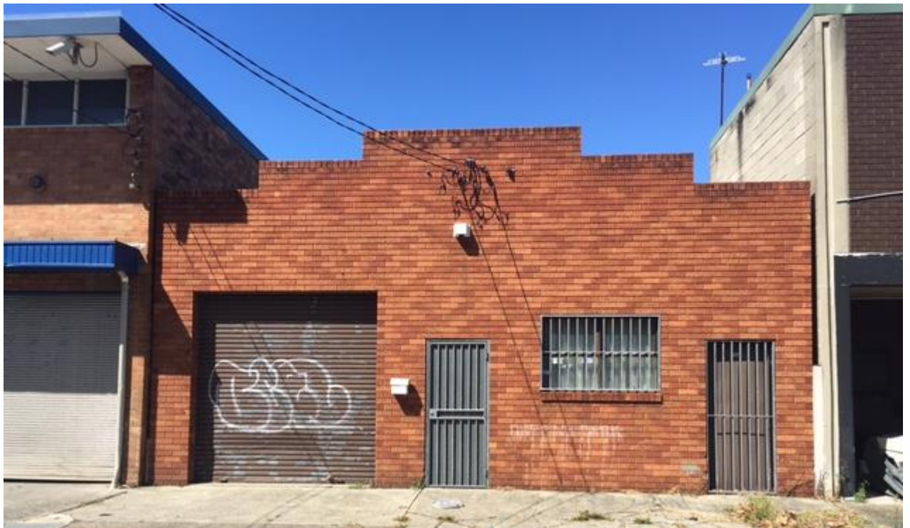
13 FAVERSHAM STREET (EAST) – CITY STAGING STORAGE
