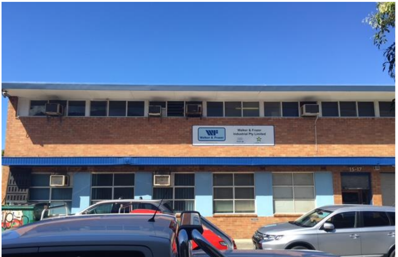
15-17 FAVERSHAM STREET (EAST) – G WALKER & FRAZER ELECTRICAL OFFICES
